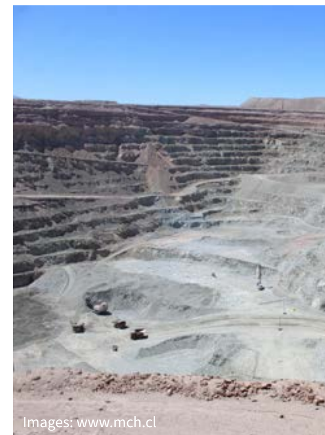
Gabriela Mistral: Located in the Antofagasta region, this operation produces copper cathodes obtained by solvent extraction and electrowinning. It is the only mine in Chile with a fully autonomous truck fleet. In 2023, it produced 105,825 tons of copper.
